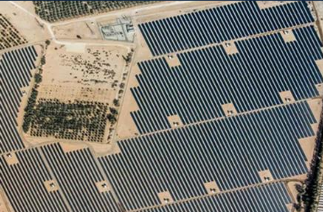
KTURA 40MWp plant
