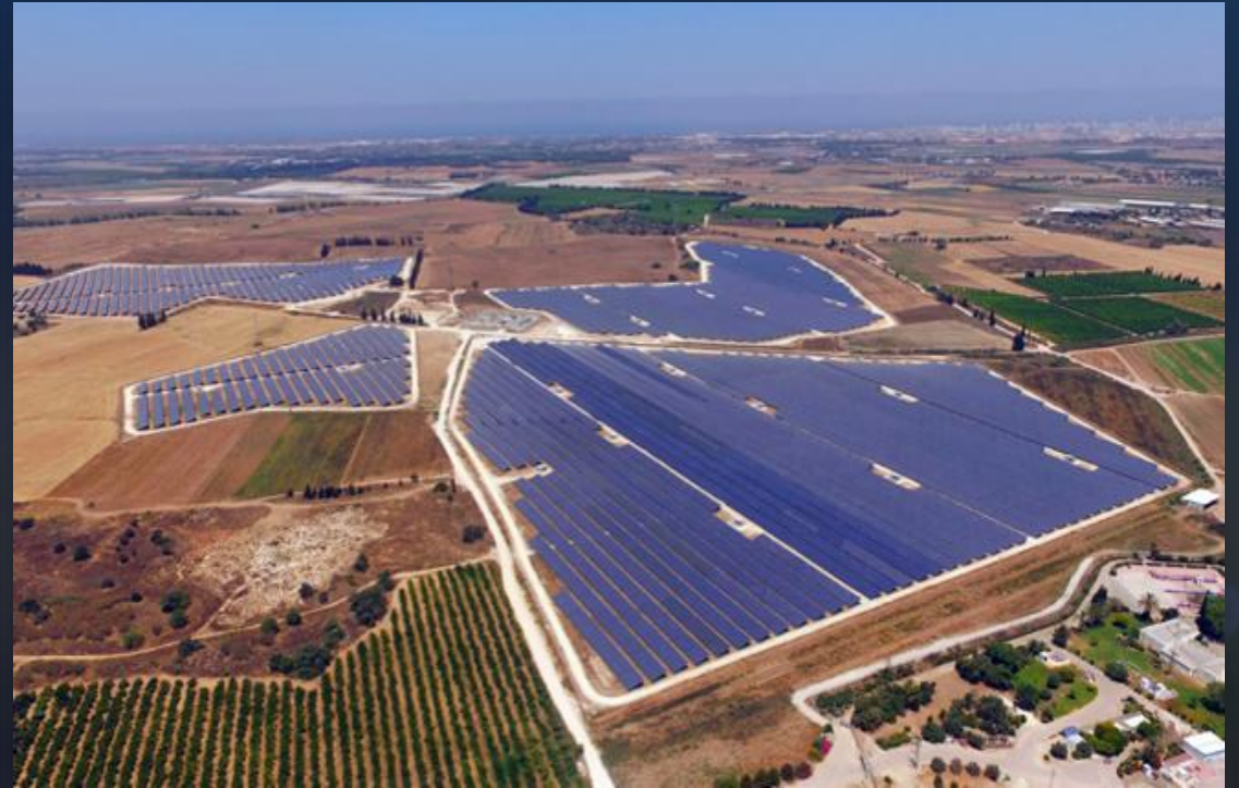
ZMOROT 50MWp plant
